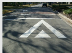
White Chevron Pavement Marking
